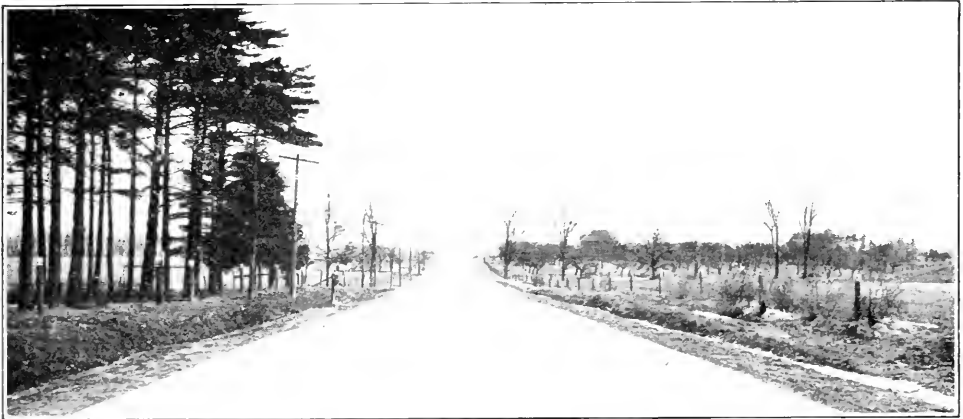
LONDON-ST. THOMAS PROVINCIAL HIGHWAY Concrete pavement constructed during 1921.
